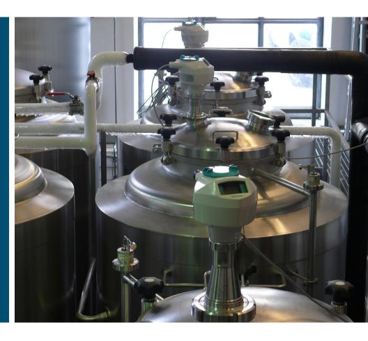
Previously, this would have been done primarily using ultrasound sensors with direct product contact, or by means of differential pressure measurement. Siemens has offered the Sitrans LR250 HEA, a system for pressure measurement without product contact, based on the technology of the cross-sector Sitrans LR250 radar level transmitter.
