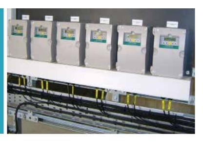
trast, the SITRANS FST020 uses patented transit-time sensors to demonstrate a consistently high accuracy of 1-2 %.
